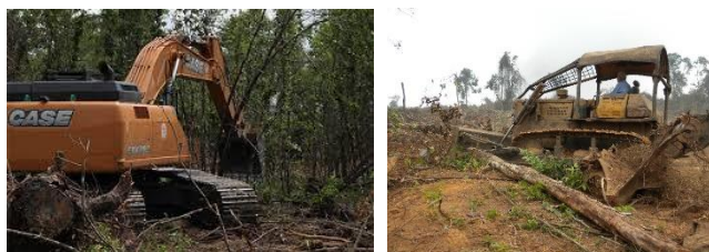
Figure 5: The use of heavy machineries during land clearing
